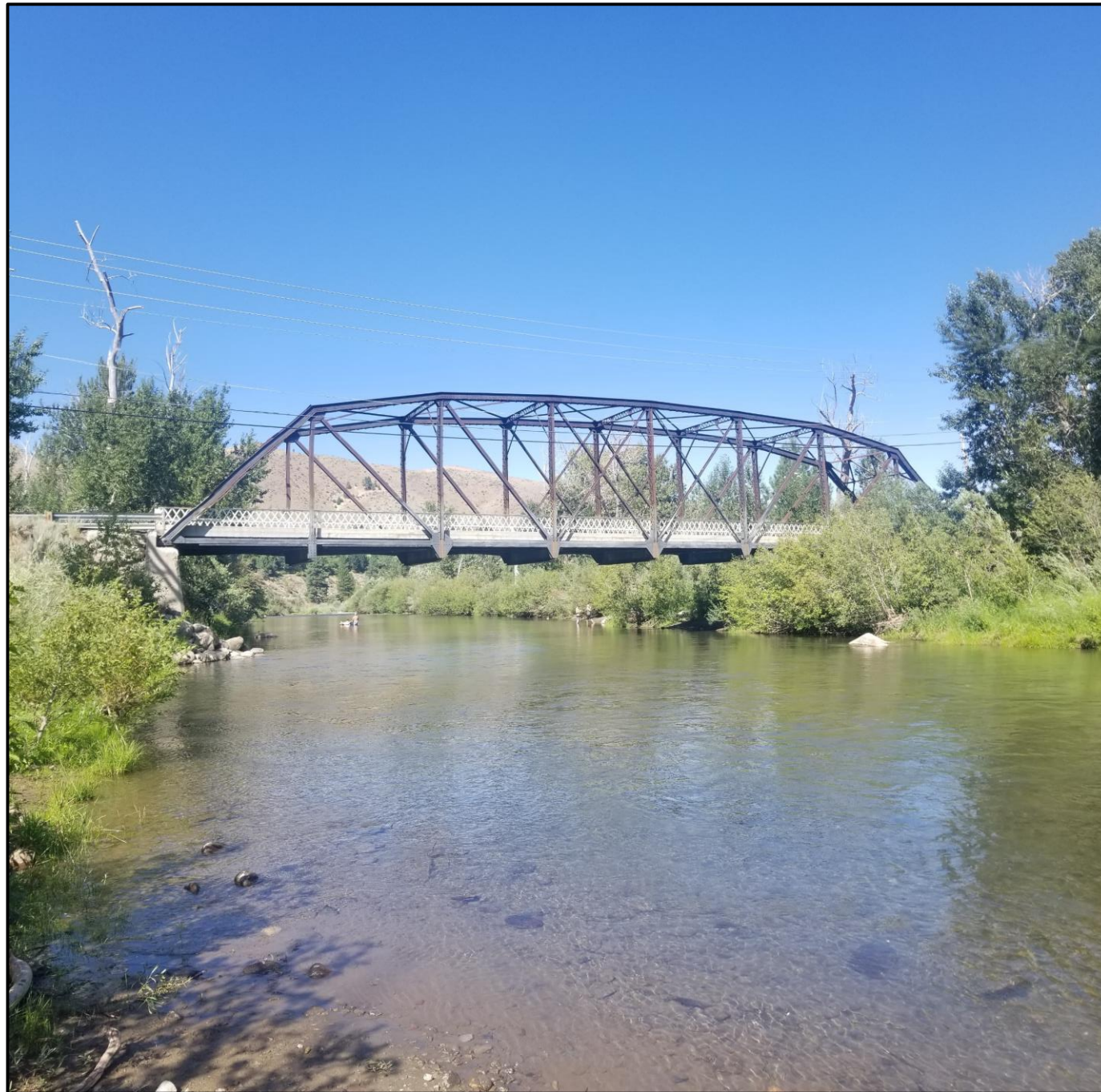
Old Steel Bridge 42.05
